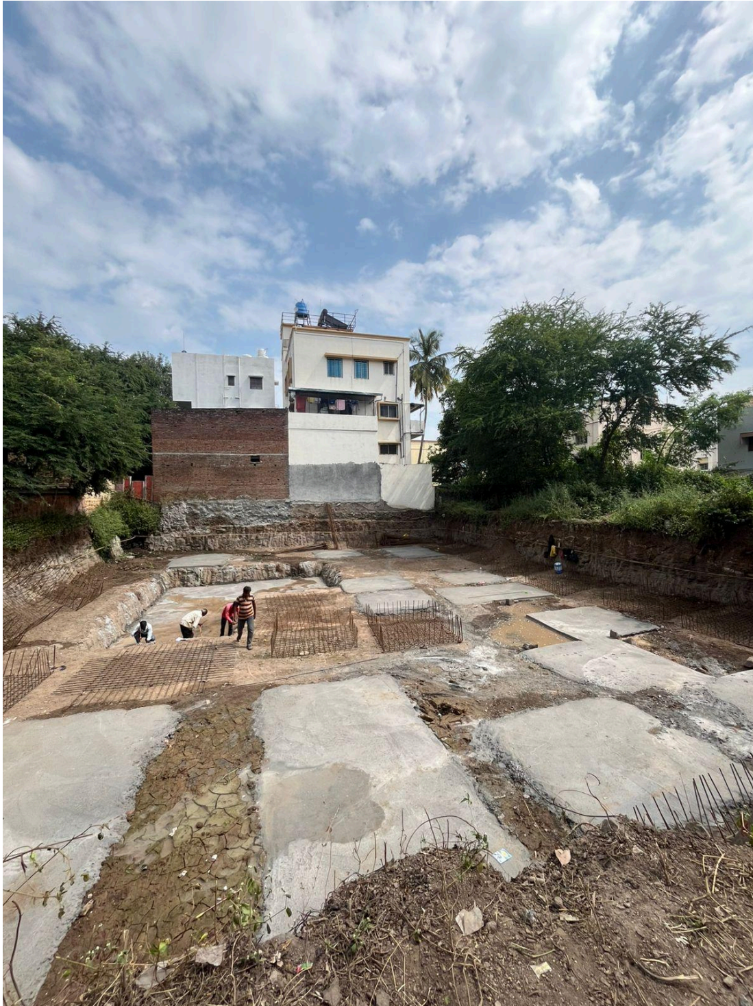
Stakeout of construction points using a Total Station, with basement excavation and footing placement underway.
