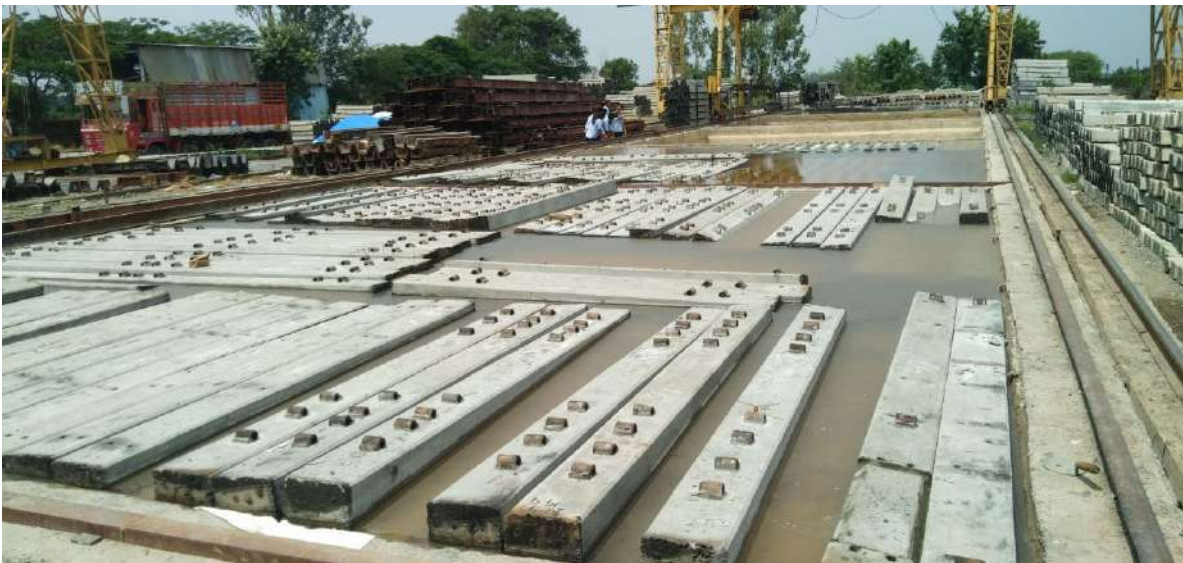
Curing of Sleepers in Rectangular Water tank
