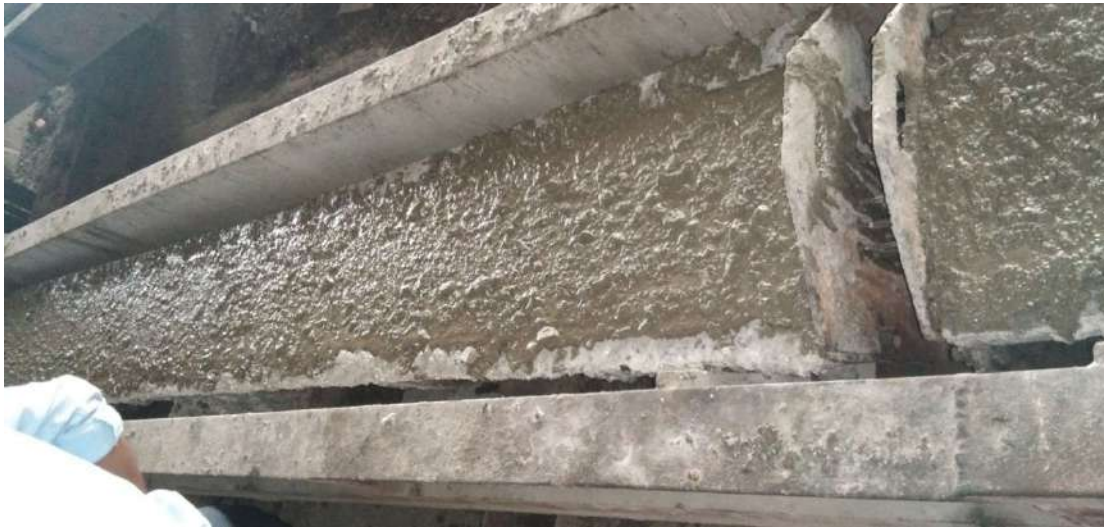
Compaction of Concrete in Sleeper Mould
