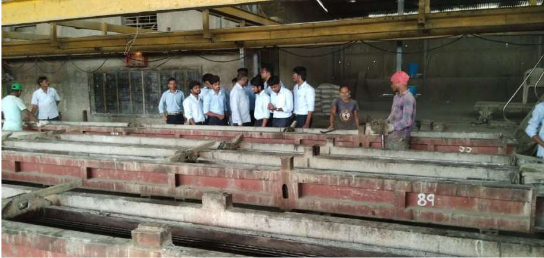
Stretching of high Tensile Steel Wires by Hydraulic Jack
